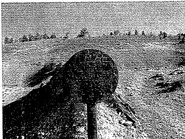
Damaged Sign between 50 and 25 yard bay note eroded lateral berm
